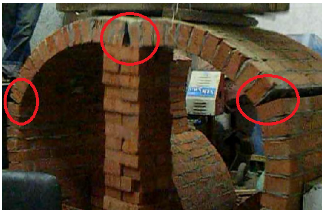
Figure 9 Control masonry vaults failure pattern.
